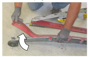
Install the rotated or new squeegee blade into the outer frame. Be sure the squeegee is completely slid down onto each tab on the outer frame.
